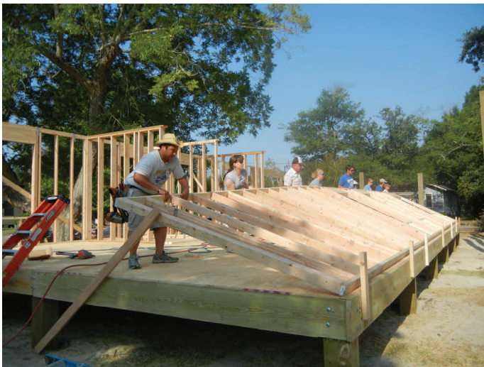
The students raise one of the walls of new home.
