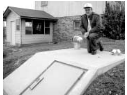
MDS Field Consultant Jim Shelly kneels on top of an underground safe room in Mulhall, Okla. The prefabricated concrete structure has a steel door and roof vents.
