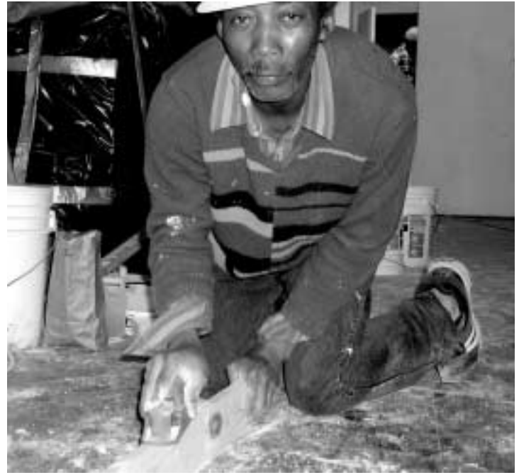
Felix Solano planes the edge of a piece of baseboard for the food pantry at the Evangelical Garifuna Church.
